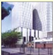
Nagarjuna Construction Company Limited (NCCL) for $150 million, one of the largest-
